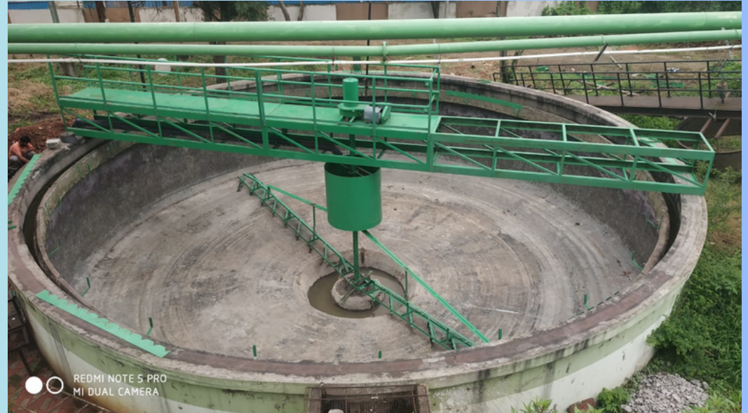
Secondary Clarifier provided at Bajaj Auto Ltd. Akurdi
