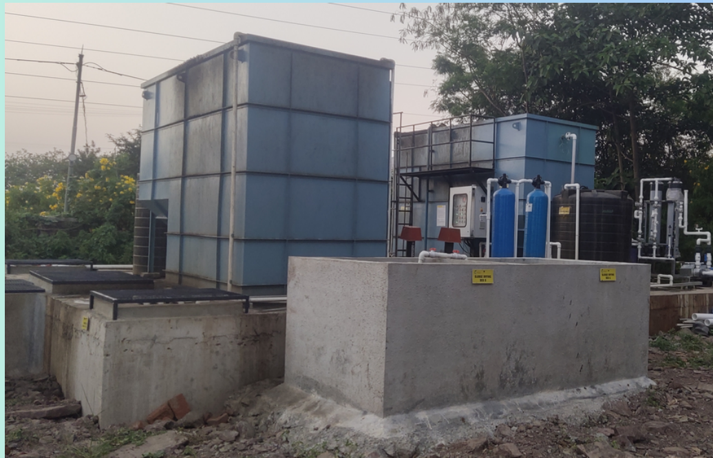
Turnkey project: 100 KLD ETP & STP- MBBR Technology Magna Automotive India Pvt. Ltd
