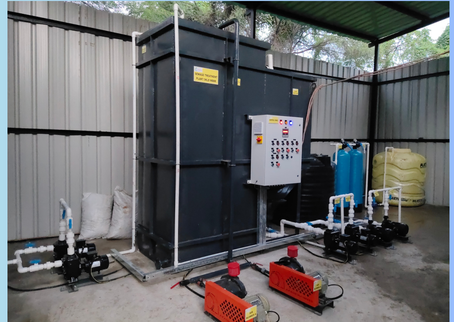
20 KLD STP: MBBR Technology at Coal INDIA
